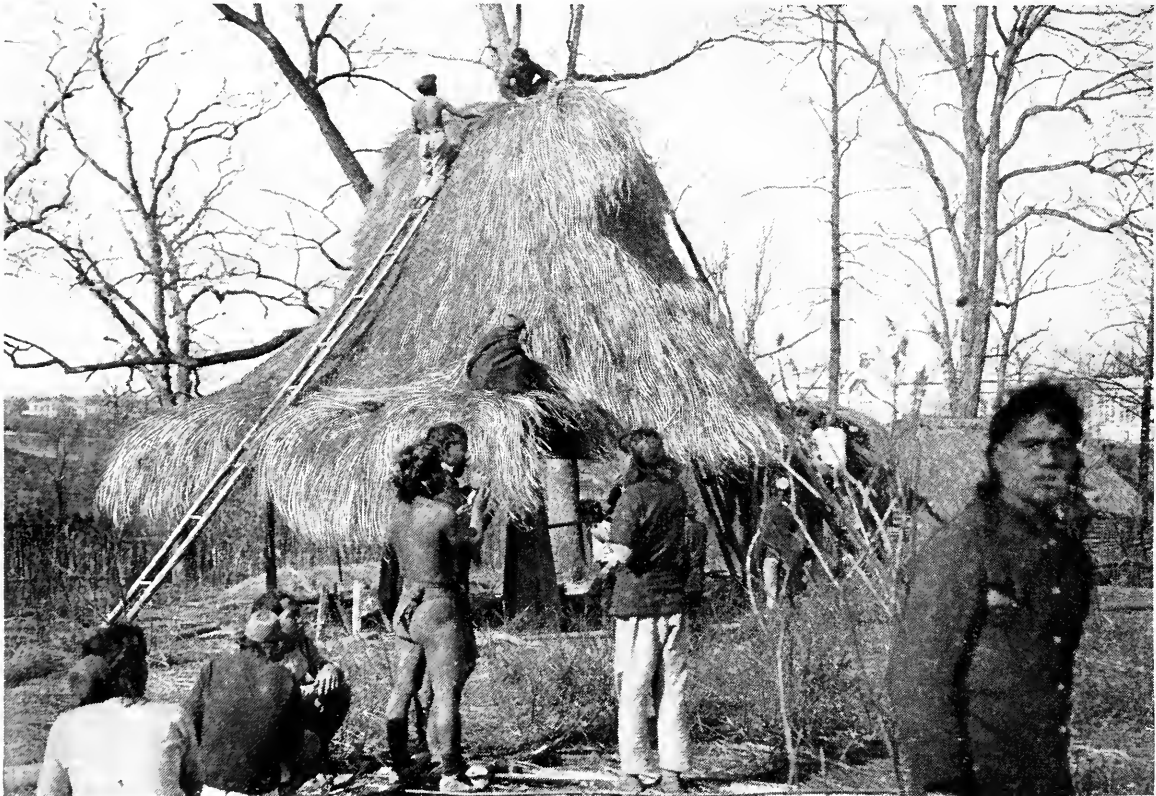
BOUTOC IGORROTES BUILDING A HOUSE
